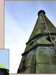
A head for heights is definitely needed here as repair work gets under way and a new lightning conductor is fitted. Pictures taken by LPS.
